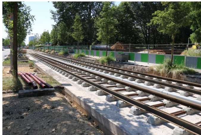
Figure 15: Chantier Tram à Kirchberg, source: Luxtram S.A.
